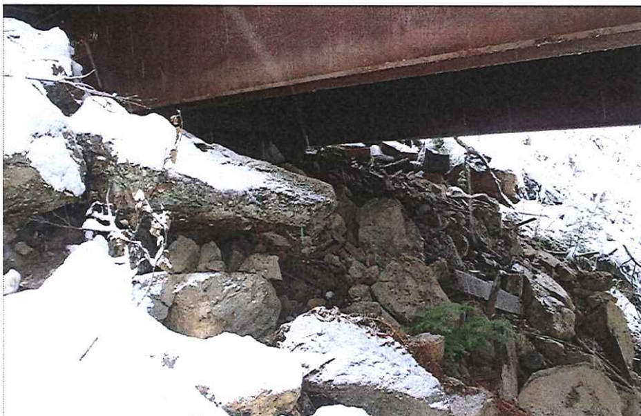
CK2279 Left Abutment
