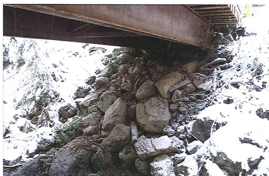
CK2279 Right Abutment
